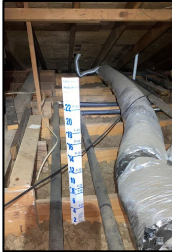
Pre-install Representative Area
