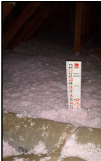
Post-Install Representative Area
