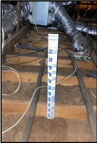
Pre-install Representative Area
